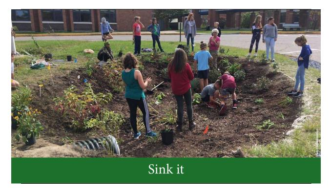
At Shelburne Community School, this project transformed the area in the middle of the school bus circle from a grassy lawn with storm grates (where water went directly from the parking lot into McCabe's Brook) into a rain garden, which allows the water to sink into the ground, getting cleaned up by the plants in the rain garden before being sent on to the brook and lake.
