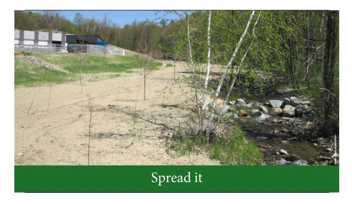
At this site, the Hinesburg Town Garage, buildings and a berm next to Beecher Brook were removed, to make space for the stream to spread out onto what was originally its natural floodplain, but had been filled in over time. In addition, rocks and logs were added to the brook to raise its level, to allow it to spread out onto its new floodplain, thereby dropping sediment held in the water before it gets washed down the brook to the LaPlatte River and Lake Champlain.
