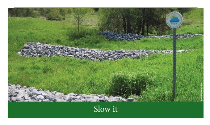
This site, E. Thompson's Point Road in Charlotte, is a roadside swale designed with these rock check dams to slow water down before it drains into Thorp Brook.
