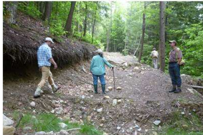
8. Forest road installed across >35% slopes, to access patch cuts. Steepness of hillsides and use of skidders necessitated wide road cuts. Steepness of road grade (>10%) required frequent water bars.
