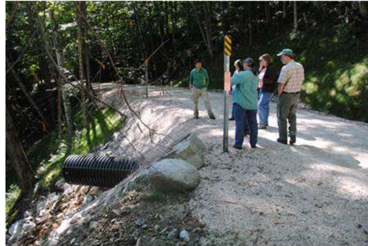
2. View downhill, same culvert site as photo 1.
