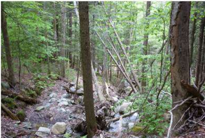
7. Incision and widening of stream channel observed downslope from C2 forest road crossing.
