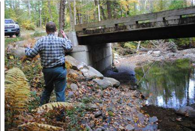
Abutment replaced after TS Irene
