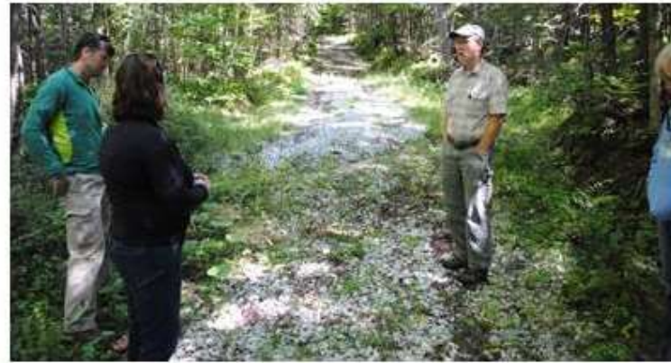
(b) broad-based dips installed on forest road in Plymsbury WMA off Old Shrewsbury Road.
