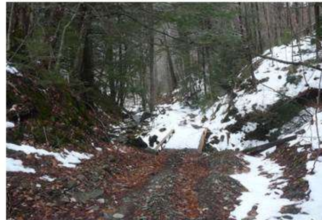
8. Road ditch directs runoff to the stream at the bridge crossing.
