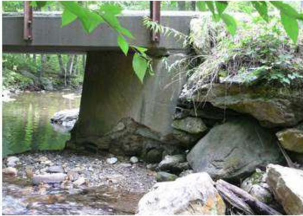
5. Right-bank abutment of Scout Camp Rd (2009)
