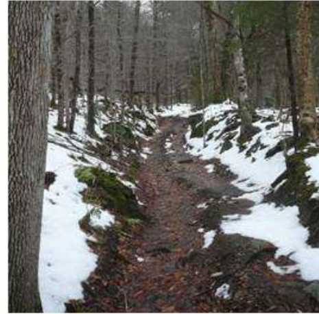
6. View uphill on narrow forest road that is channeling runoff; dugway banks are 5 ft high in sections.
