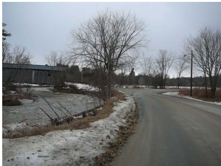
Figure 18. Berm along Spear Street upstream of Quinlan Bridge.
