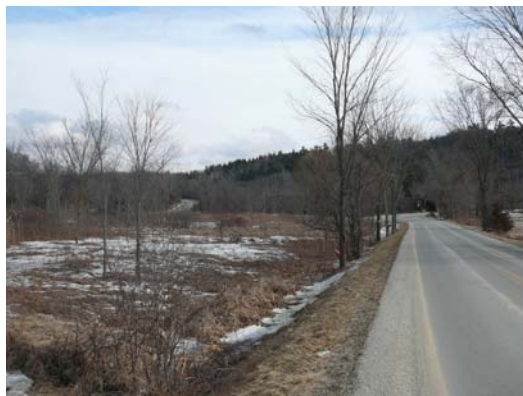
Figure 28. Spear Street west of Quinlan Bridge; view to the east toward the bridge site.
