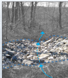
Treatment 2 Rock-lined Entry
