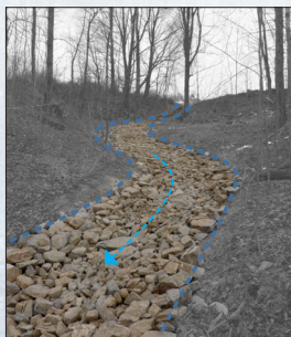
Treatment 1 NRCS Rock-lined Waterway
