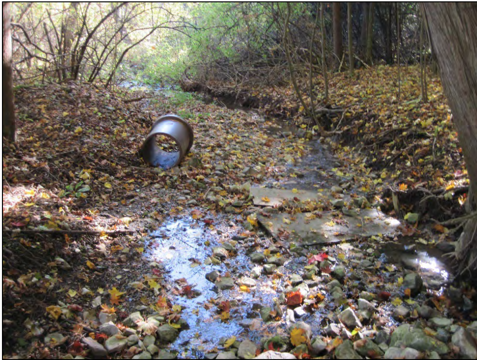
Figure 4. Intermittent stream below convergence of stone-lined swale and standpipe.
