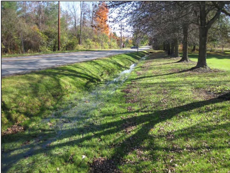
Figure 6. Grass-lined swale along Harbor Road.
