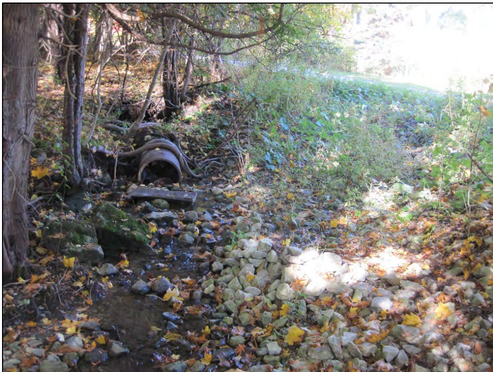
Figure 2. Outfall of standpipe and stone-lined swale turnout.
