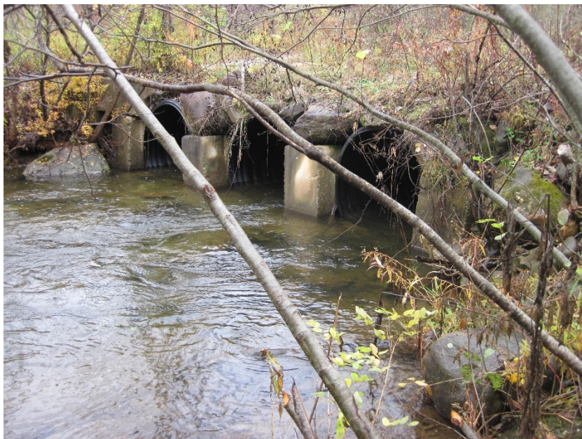
Driveway culvert viewed from upstream.
