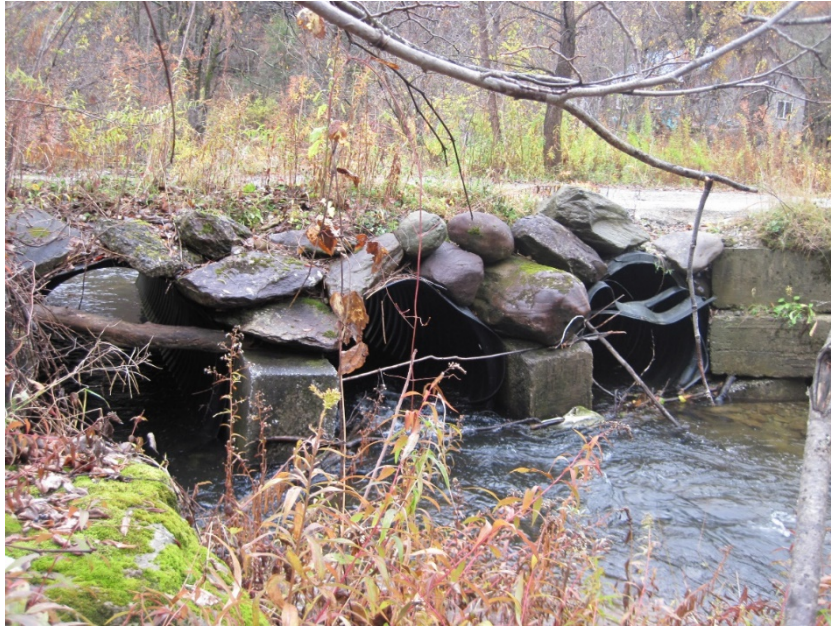
Driveway culvert viewed from downstream.
