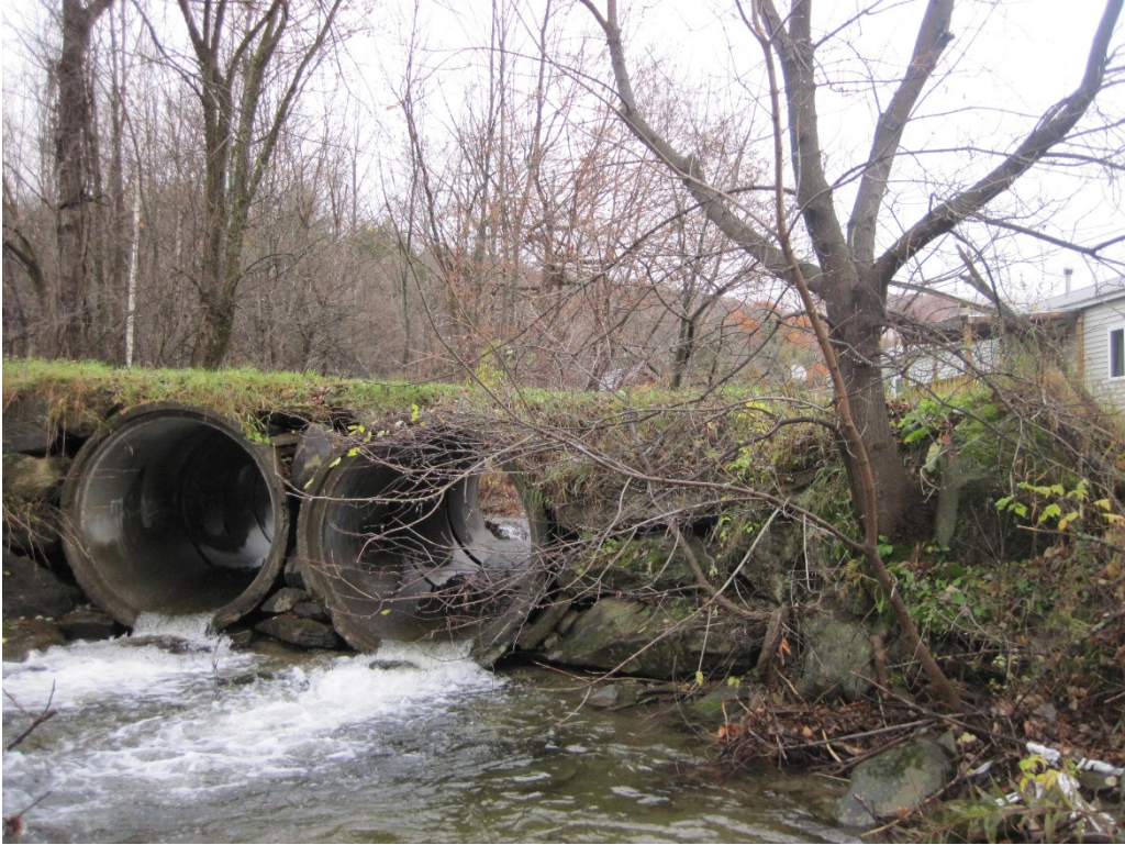
Sugar Hollow Lane culverts, viewed from downstream.
