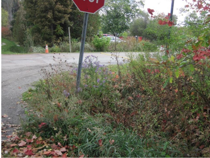
Photo 2: Culvert under Lyman Meadows Road (Project #2).
