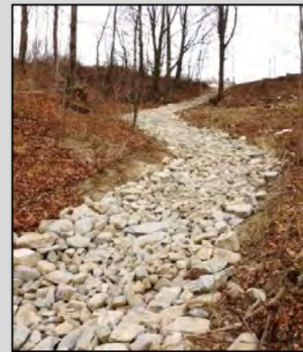
Figure 1. NRCS Rock-Lined Waterway practice installed to stabilize Gully #3, Jan 2015
