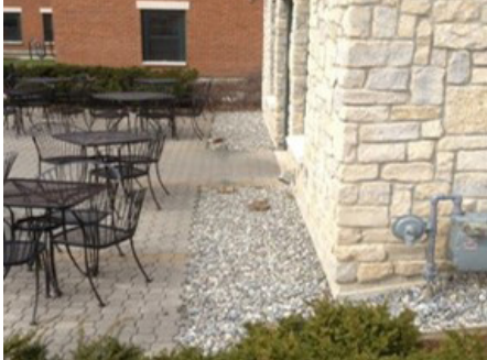
INFILTRATION TRENCH. Filters and infiltrates runoff in existing flow paths, along walkways and driveways, or in the drip line of non-guttered roofs.
