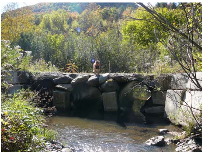
Figure G-64. Triple-culvert driveway crossing of Hollow Brook at 1237 Hollow Rd at the upstream end of Segment T4.02-B. Reinforced with boulders and concrete blocks. View downstream, 10 October 2008.
