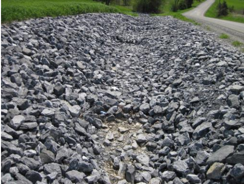
Reconstructed stone swale, East Thompson Point Road, Charlotte, Vermont, May 17, 2017
