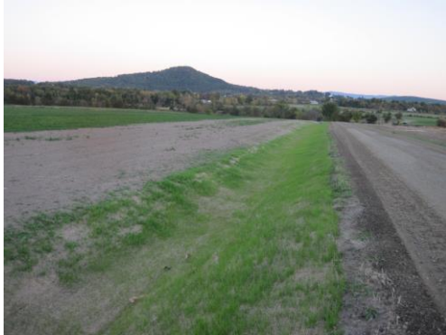
Reconstructed grass swale, East Thompson Point Road, Charlotte, Vermont, Summer 2016
