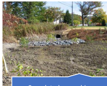
Completed upper bio-retention cell looking east
