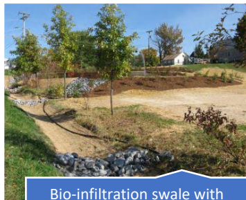
Bio-infiltration swale with stone trench example from the Silver Street rain garden
