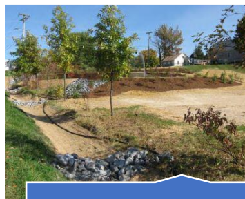
Adjacent completed Silver Street rain garden
