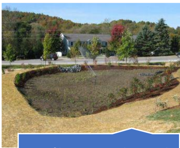
Bio-infiltration trench example from Silver Street rain garden
