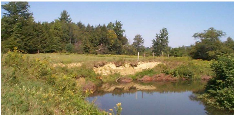
Figure 2. Meander Bend A at Clifford site (reference Map 1). (Above) - meander in August 2001 exhibiting active slumping and erosion; note cedar revetments along water line. (Right) - meander in May 2005, erosion mostly healed.
