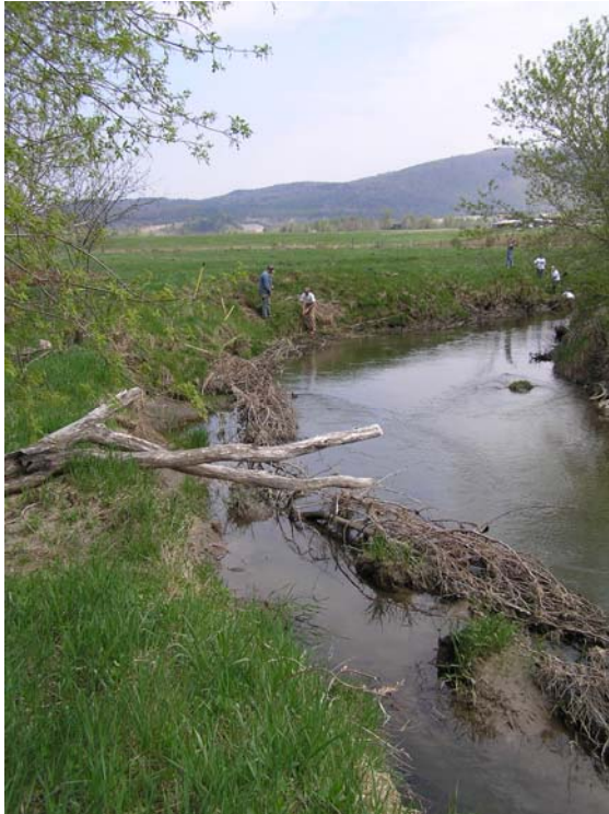
Figure 4. View upstream from Meander B in Map 1 (May 2005). Cedar revetments along right bank (facing downstream) installed in 2003 were laterally outflanked. Background: volunteers installing willow waddles along top of cedar revetments.
